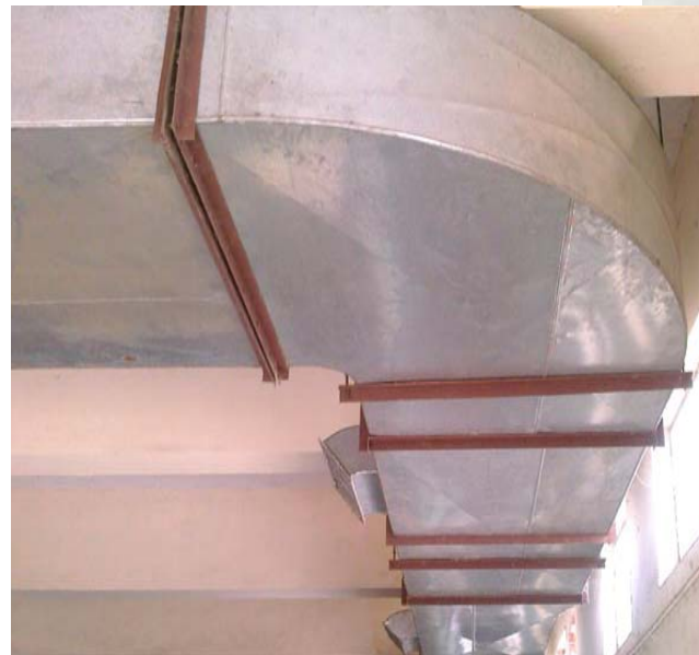
DUCT DISTRIBUTION AT OFFICE TO FLOW COOLED AIR
