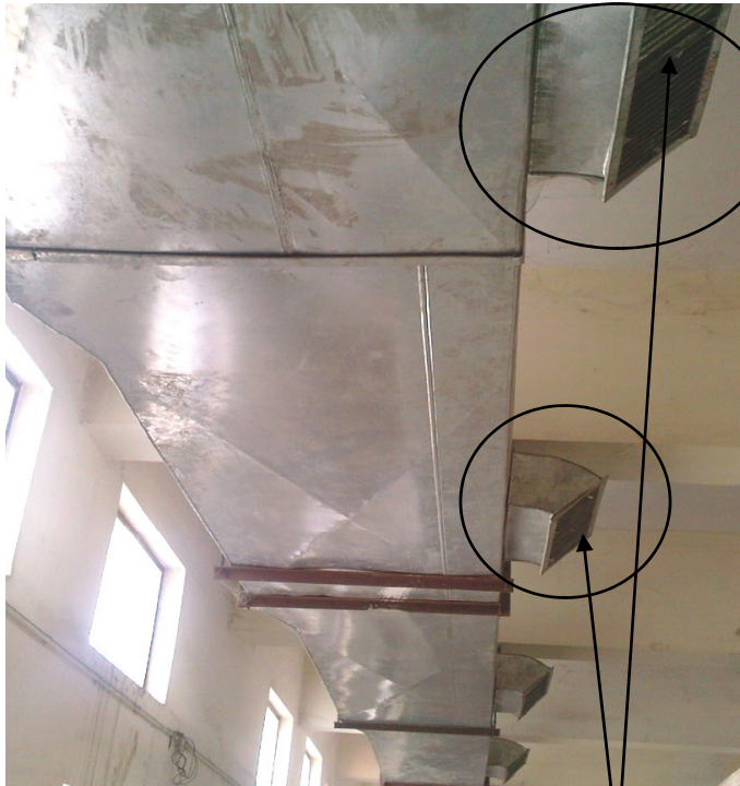
CENTRAL AC VENTILATION TO THROW COOLED AIR
